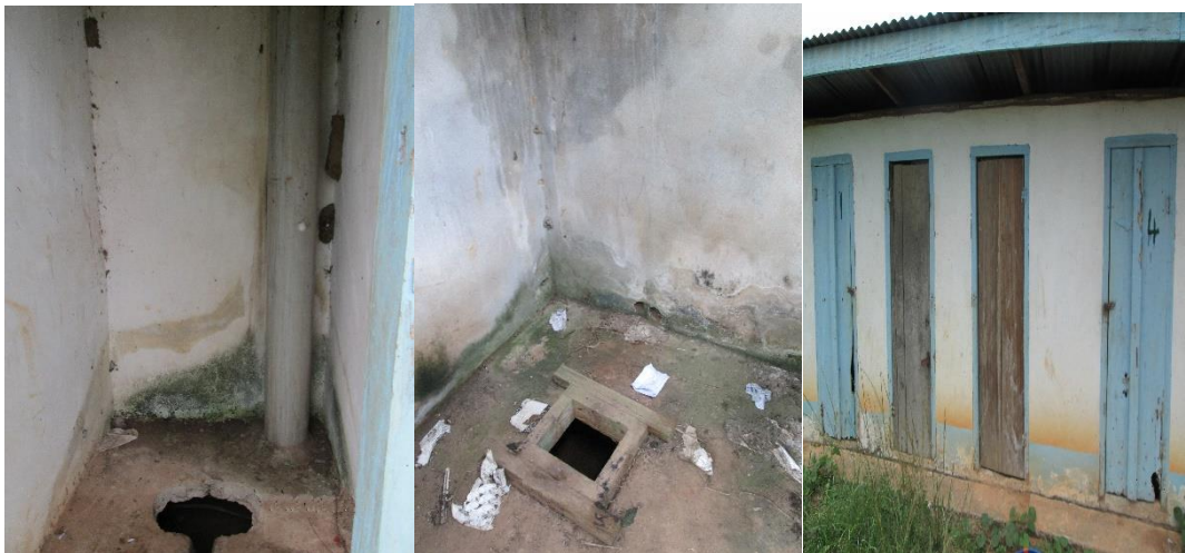
Figure 16 ULICA Mission School VIP Latrine (left), Traditional Latrine (middle), and Latrine Superstructure (right)
